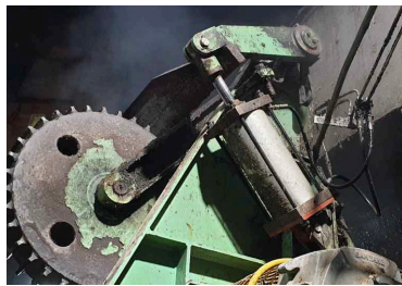
(파손 전)RAGGER WHEEL
